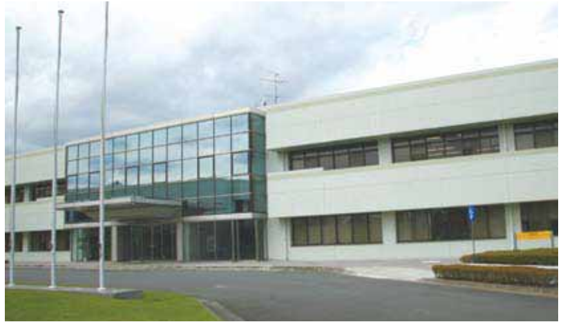
JIRCAS Main Building
