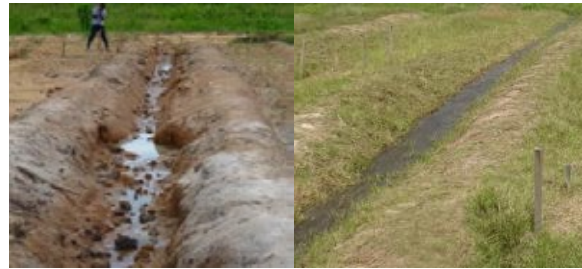
Fig. 3. Test canal 6 months after installing. Left: Canal without vegetation Right: Canal planted with ground covers
