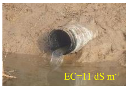
High-salinity leach water is discharging into an open ditch.
