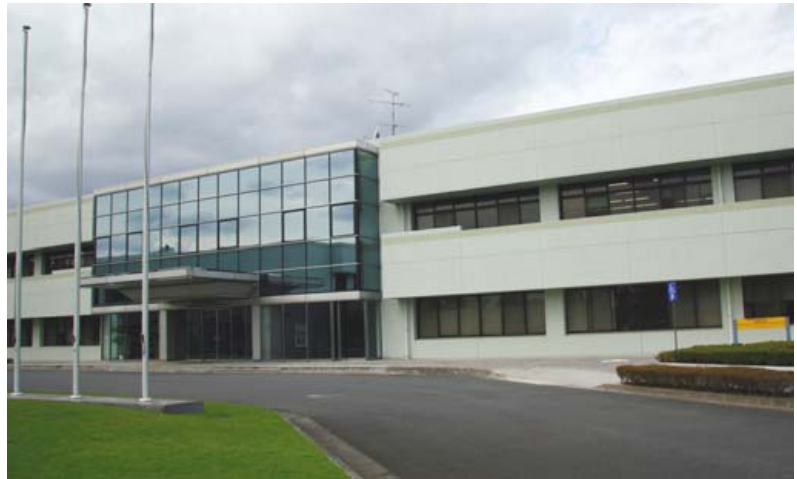
JIRCAS Main Building
